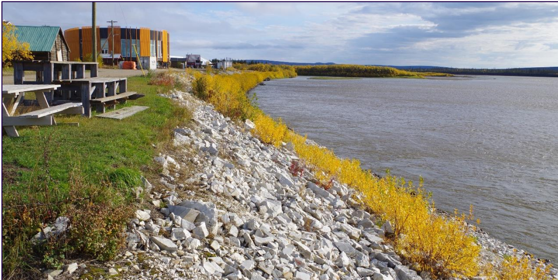
FIGURE 6.1.1. EROSION PROTECTION ALONG THE PORCUPINE RIVER IN OLD CROW LOOKING EAST
